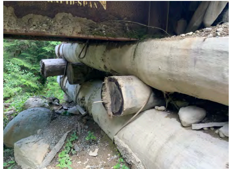
Right Bank Abutment when facing downstream
