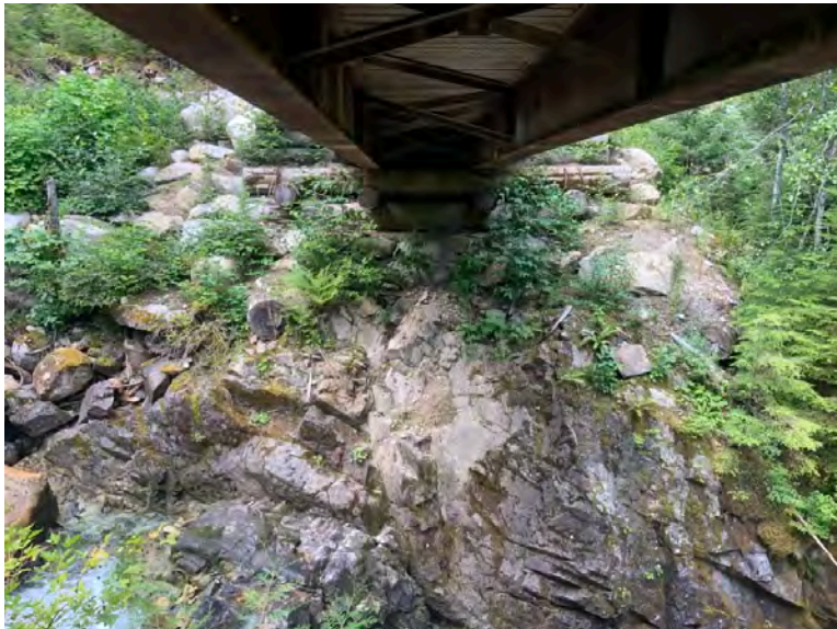
Left Bank Abutment when facing downstream
