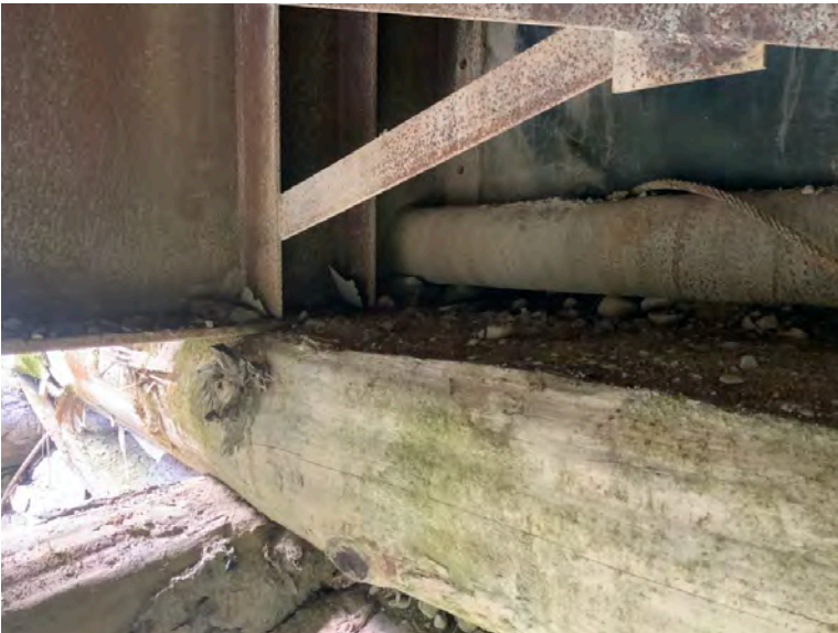
Left Bank Abutment when facing downstream
