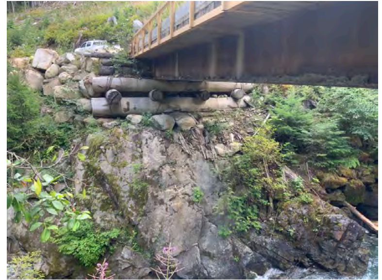
Right Bank Abutment when facing downstream
